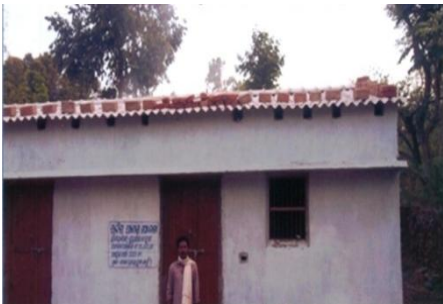
IAY House in Ballam GP of Barkote Block
