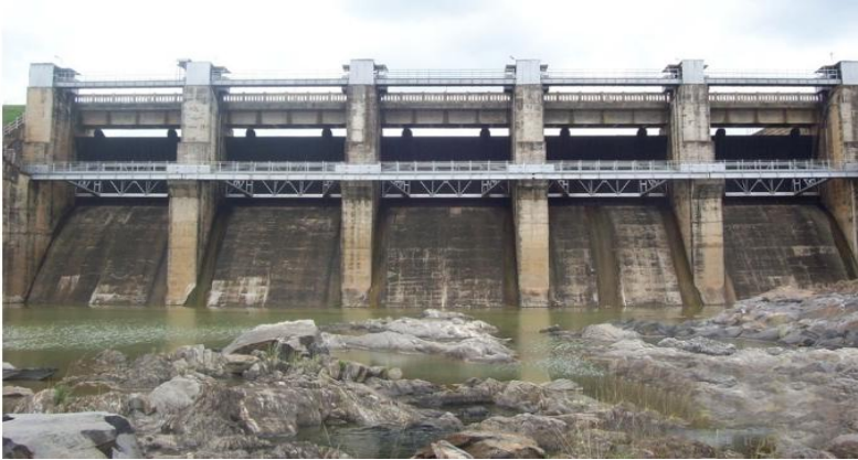
A view of the Gohira Dam from the riverbed
