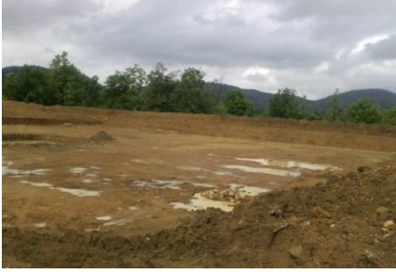
Fish farming tank under construction
